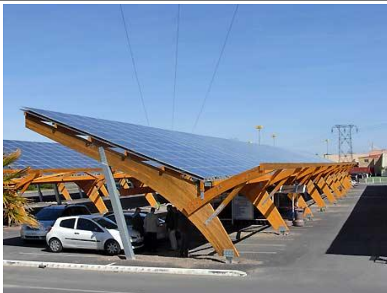
Figure 53: Ombrière photovoltaïque
